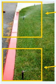
Old sprinkler spraying water onto the driveway.
